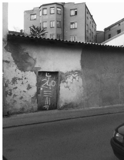
Fig. 11. Rectangular shaped house with one opening, Hercegovačka street, Belgrade
