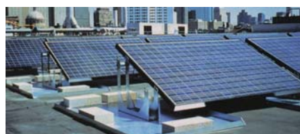
Fig. 1a. Roof "standoff" PV system
