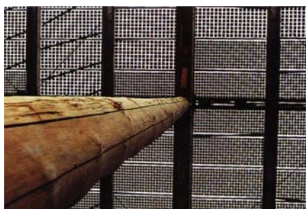
Fig. 5. Light permeability produced through the variation of the arrangements and distances between the PV cells; a) facade permeability,
