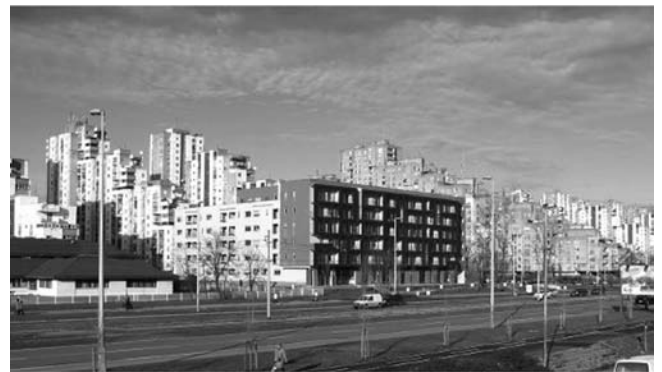
Figure 3. Group I-B, Social non-profit housing in PFC 10, Jurija Gagarina Street, Block 61, New Belgrade
