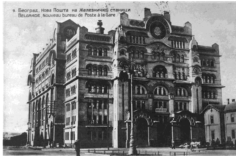
Figure 1. Momir Korunović, Post Office Building 2, 1928. (scanned postcard, personal archive)
