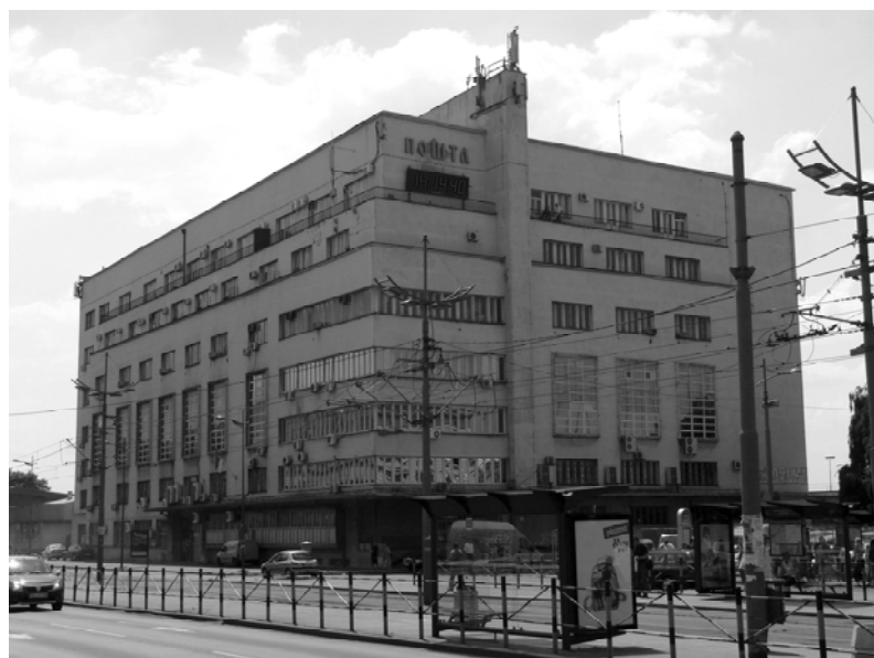
Figure 2. Pavle Krat, reconstruction of Post Office Building 2, 1948.
