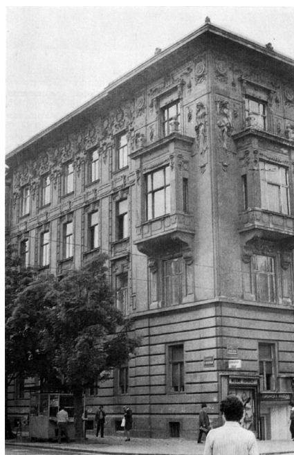
Figure 2. Art Nouveau façades of the Rado rental apartment house (Source: Živković, 1977)
