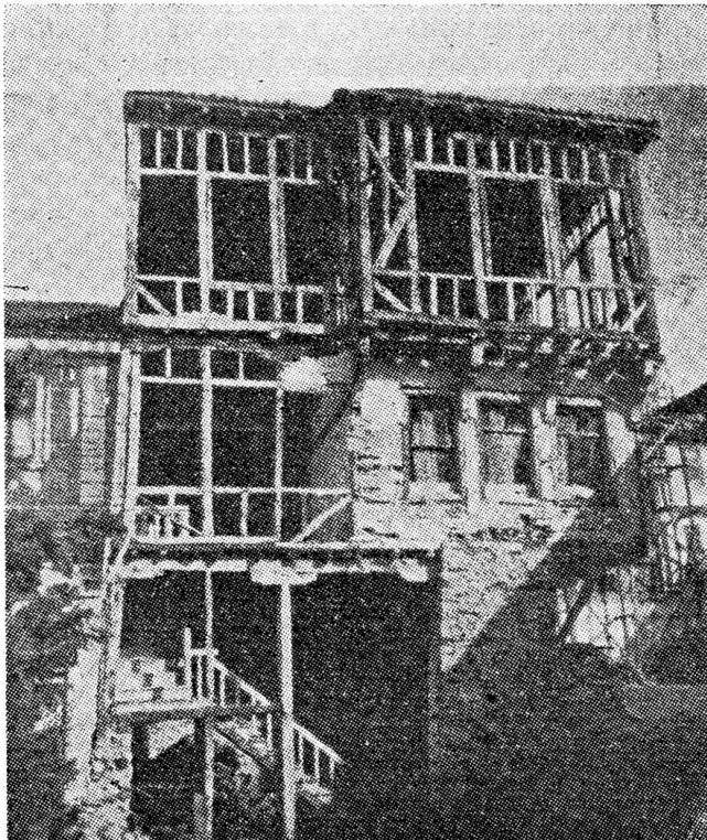
Figure 1. Skeleton of a wooden bondruck system at a house in Ohrid (Source: Tomovski, 1959-61: 3)
