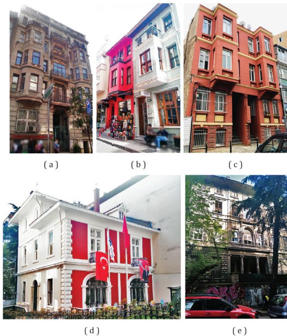
Figure 4. Examples of housing typologies from the selected site, which still exists today (a) an Armenian apartment – Demirciyan Apartment – in Yeldeğirmeni; (b) Greek houses in Caferağa; (c) a Jewish house in Yeldeğirmeni (source: Olgar, 2021); (d) a Levantine house in Moda; (e) a Turkish konak in Moda
