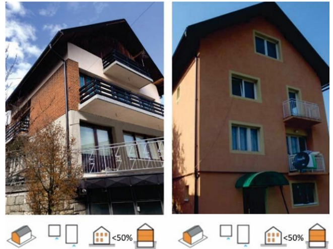
Figure 6. The second house type and a similar house from the Atlas of Family Houses of Serbia (Source: left image is by the author and the right image is from Jovanović Popović et al., 2012b)
