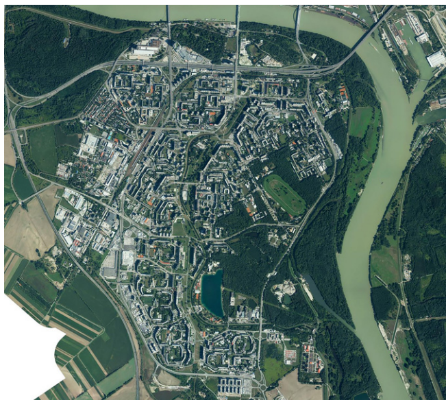
Figure 2. Mass housing structure of Petržalka (Source: GKÚ / NCL, 2020)
