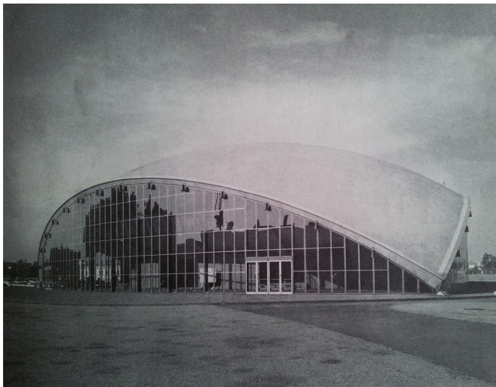
Figure 4. Auditorium of the Massachusetts Institute of Technology in Cambridge (USA), 1954-1956. Eero Saarinen, calotte-shaped shell on three supports (Source: One hundred years of significant building (1956). 6: Public Assembly , Architectural Record , November 1956, Vol. 120, No. 5, pp. 197-200)
