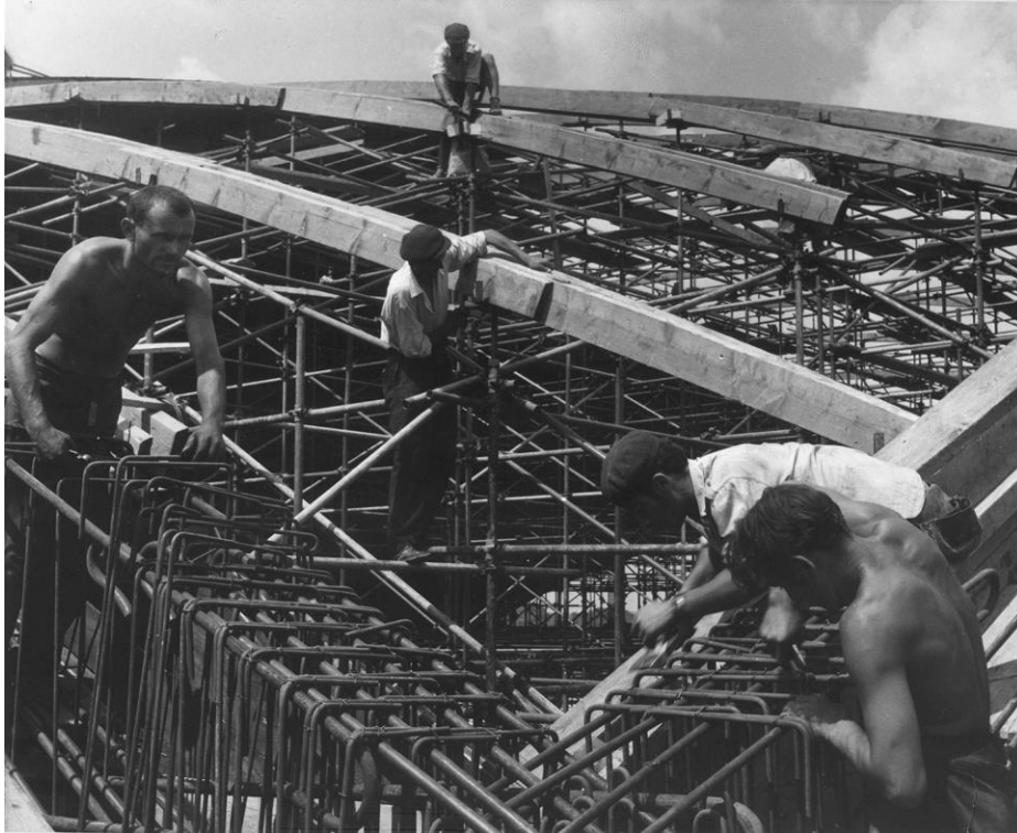
Figure 7. Construction of Hall 2 of the Belgrade Fair – assembly of the rebar for the edge arches and the structure of the shell (Source: https://sajam.rs/sanu-izlozba-posvecena-fenomenu-beogradskog-sajma-ulokalnim-i-svetskim-razmerama/# )
