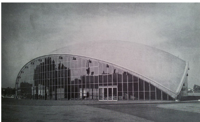
Figure 4. Auditorium of the Massachusetts Institute of Technology in Cambridge (USA), 1954-1956. Eero Saarinen, calotte-shaped shell on three supports
