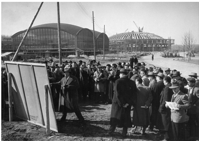
Figure 3. Construction of the Belgrade Fair – a view of Halls 2 and 1 and the park
