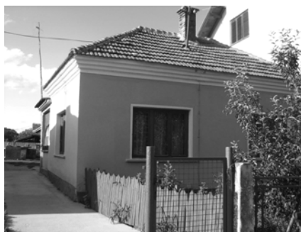
Figures 4a. and 4b. Representatives of the least (a) and the most (b) common individual housing unit types in East Serbia region (statistically): (a) a house built after 2001 (b) a house built between 1946 and 1970
