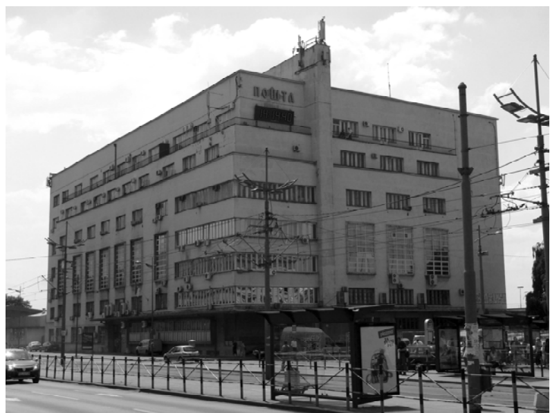
Figure 2. Pavle Krat, reconstruction of Post Office Building 2, 1948.
