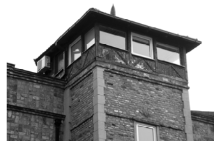
Figure 7. The combination of wood and brick as a facade lining, Milovana Marinkovića Street, Voždovac, detail of the building – the tower covered with wood (Ivanović-Šekularac, 2010)
