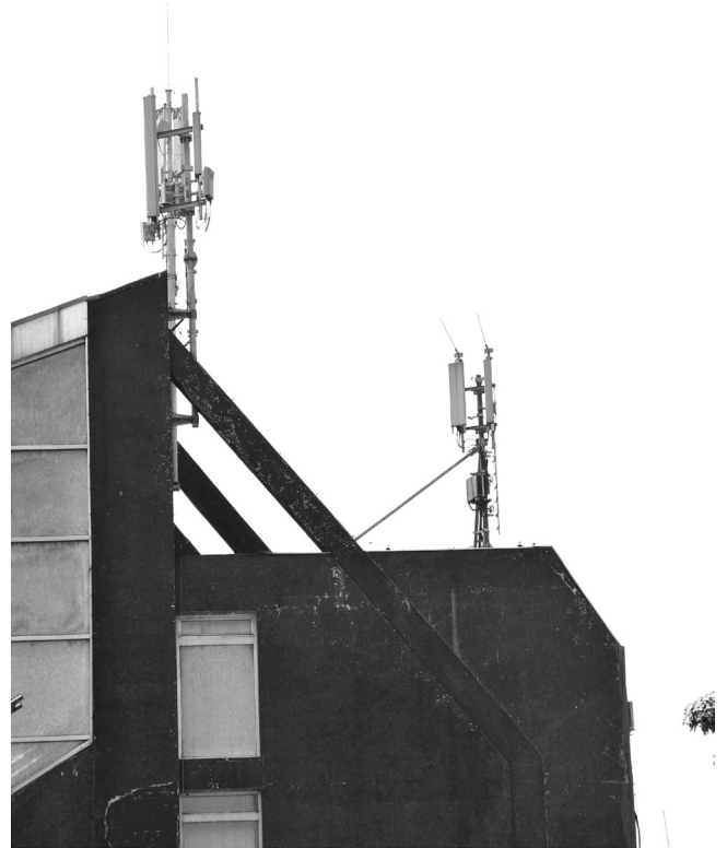
Figure 2. Detail of the main facade (Source: author)
