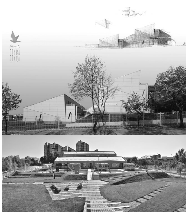
Figure 10. "Blue Bird" kindergarten, Belgrade, 2009-2011 (Source: The documentation of Milenija Marušić)
