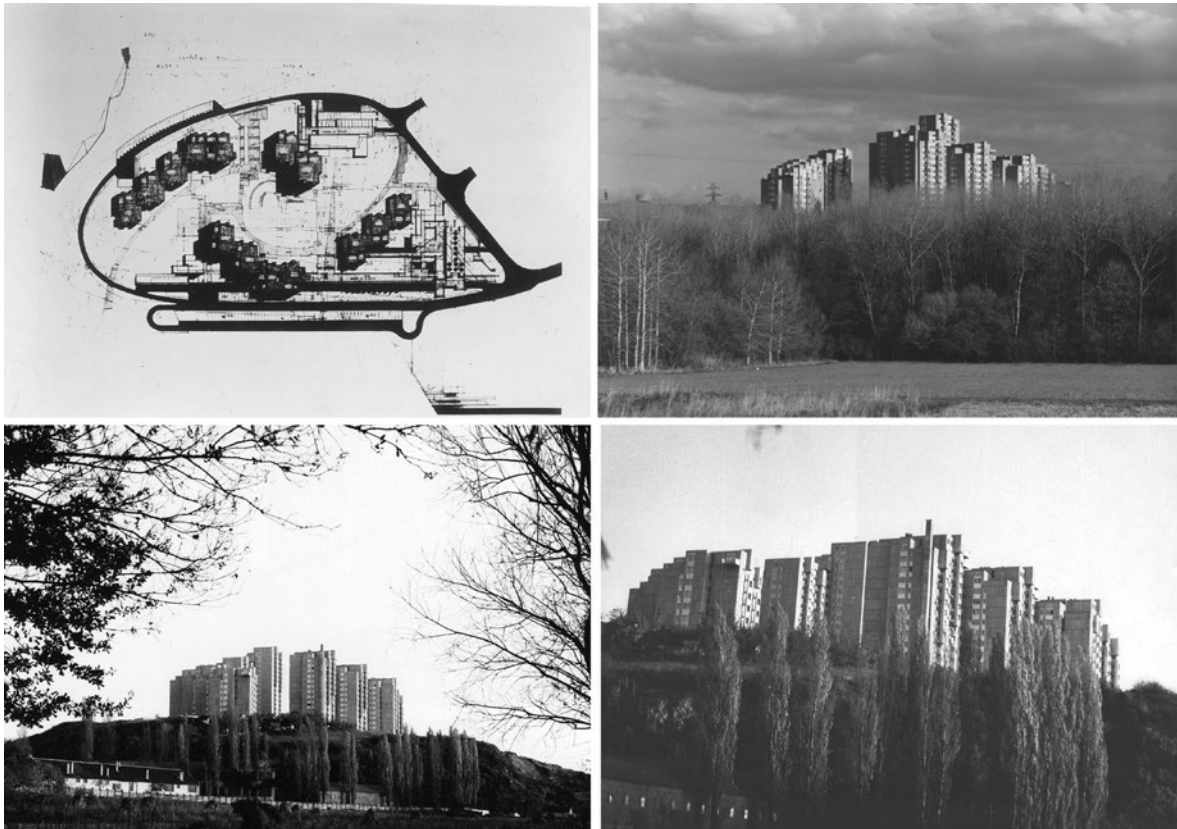
Figure 3: Milan Lojanica, Julino brdo settlement (1967-1970). Situation and photographs. (Source: courtesy of author, Milan Lojanica.)
