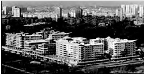
Figure 8. Overview of Type 4 - "Delevelling on the concrete"; subtype: Fortress segregation/Super-block 12 (Source: http://ilicd.tripod.com )
